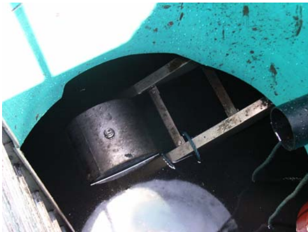
Pivot float being installed in In-Ground Interceptor
