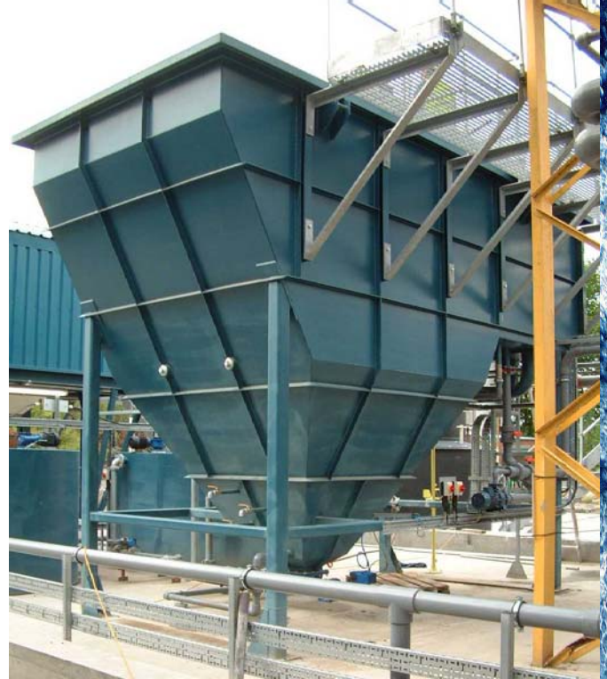
Stetmella SM75 settler with integral chemical mixing tank and clarified water discharge tank.
