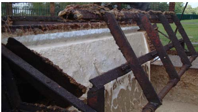
Typical surface scum from food processing effluent
