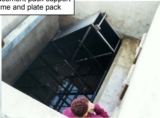
Replacement plate pack being lowered into position
