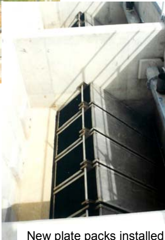
New plate packs installed
