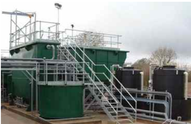
Stetmella SM75 settler with integral chemical mixing tank and clarified water discharge tank.
