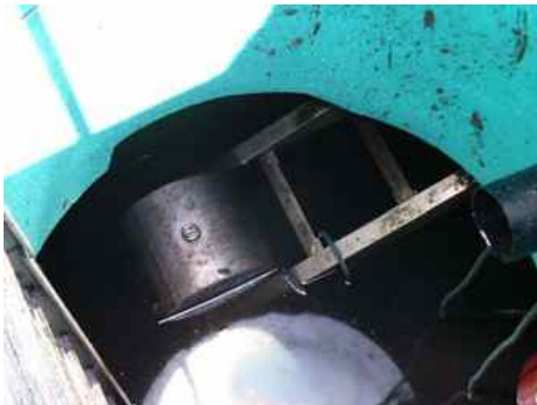
Pivot float being installed in In-Ground Interceptor
