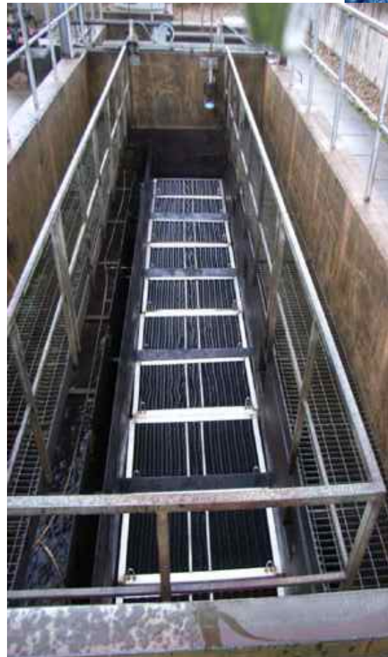
In-ground system with Polypropylene plates housed in stainless steel casings
