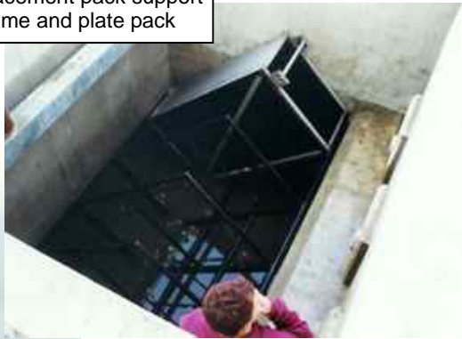
Replacement plate pack being lowered into position
